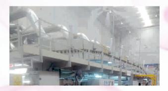
Working environment air has to recover its relative humidity by water or steam injection to the ambient. Provision of some amount of fresh air to the working environment should also help to improve productivity and to have healthy ambient. Recommended humidity level for working environment is around 55%rh.
