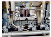
A proper condensate drainage system is essential to have a satisfied operation. Improper steam trapping should extend start-up period and should cause water hammer. Condensate flooded inside the heating plates would reduce heat transfer rate which would have negative effect on humidification efficiency.
